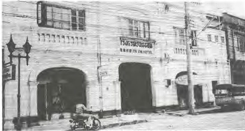
The imposing facade of the On-On Hotel.
